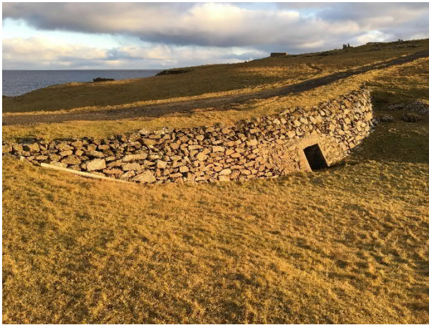
Photograph 14 – Built-up section of access track
