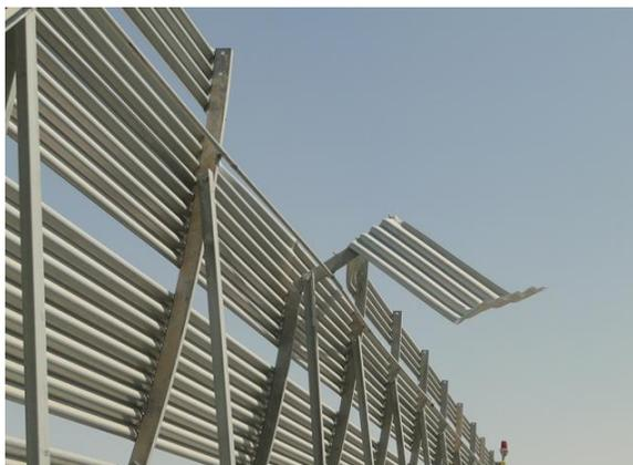
Figure 6. Damage to blast fence
