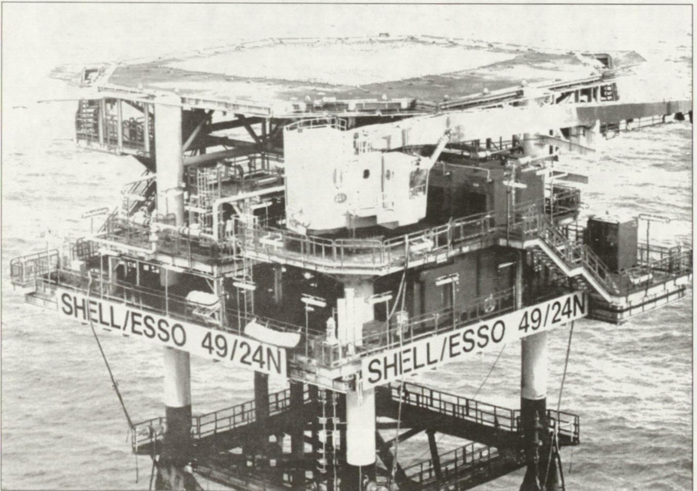
Figure 2 Rig Identification Signs
