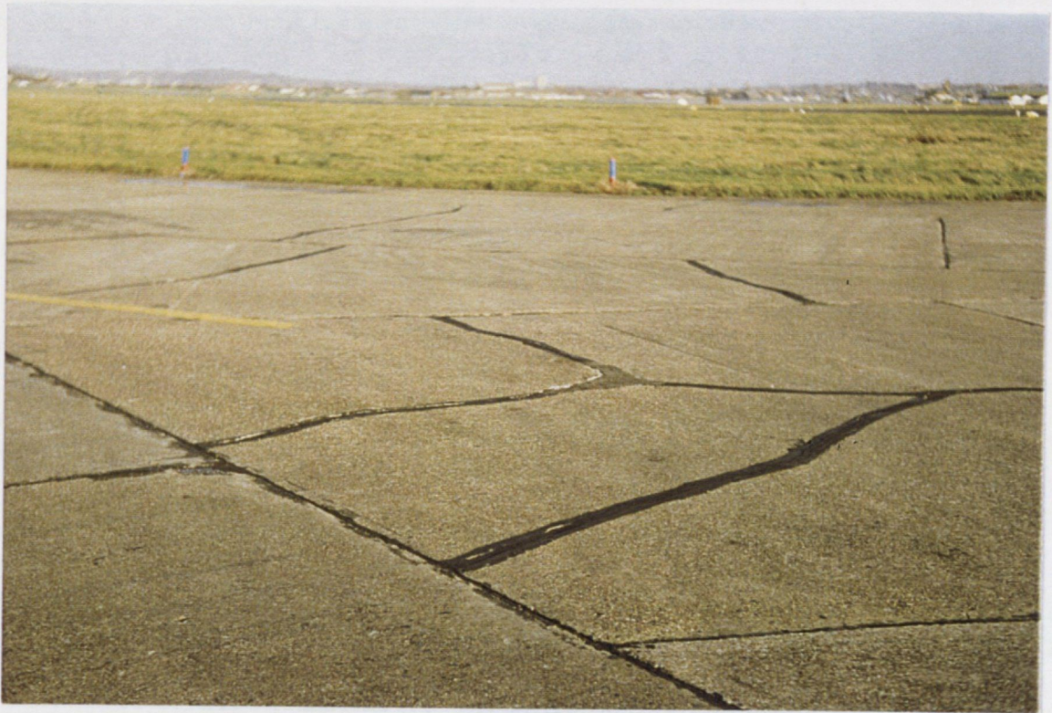
Figure 31 Extensive cracking in a rigid pavement. Pavers can be used as an overlay providing the cracks and joints are sealed and none of the concrete rocks
