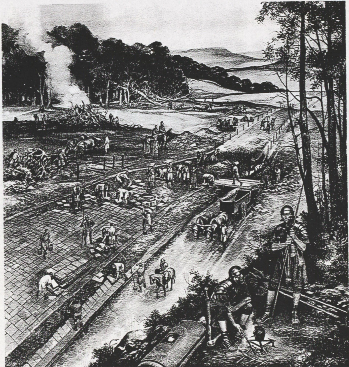
Figure 1 Roman road under construction circa 100AD in Northern England. Many of the features incorporated in present day pavement construction are in evidence: a durable paved surface, a structure sufficiently strong to withstand anticipated use, a firm foundation, edge support and drainage were all designed into Roman roads.
