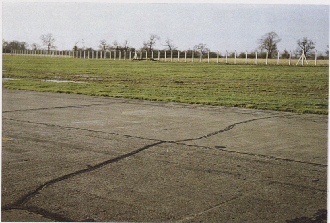
Figure 32 Transverse crack in a rigid pavement. A paver overlay is possible providing the joint has been sealed.
