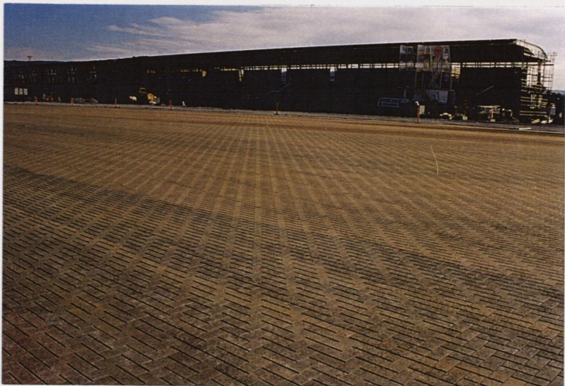
Figure 3 Herringbone laying pattern has been found to enhance the structural performance of paver projects by enhancing the interlocking nature of the pavers.
