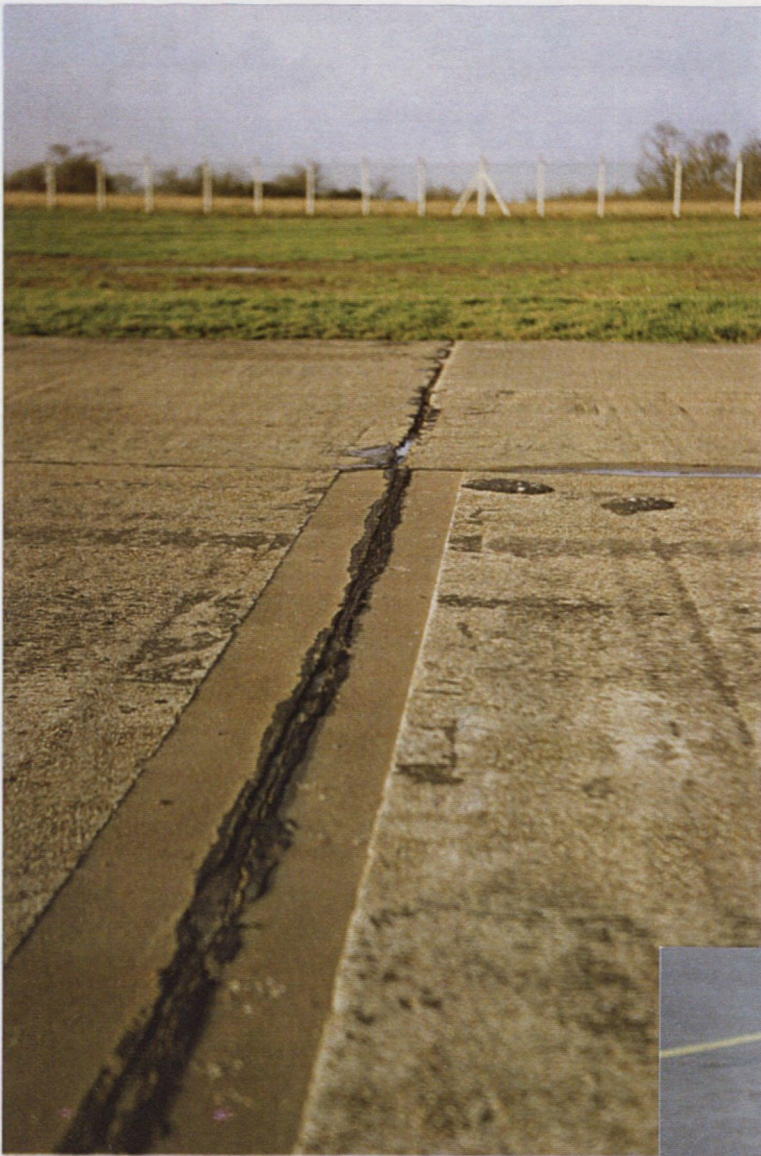
Figure 34 Reflexion crack in flexible pavement
