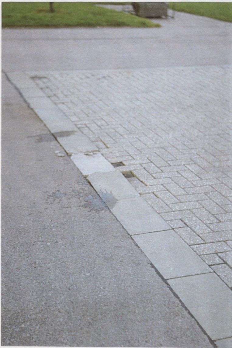
Figure 36 Spalling of edge restraint leads to Foreign Object Damage
