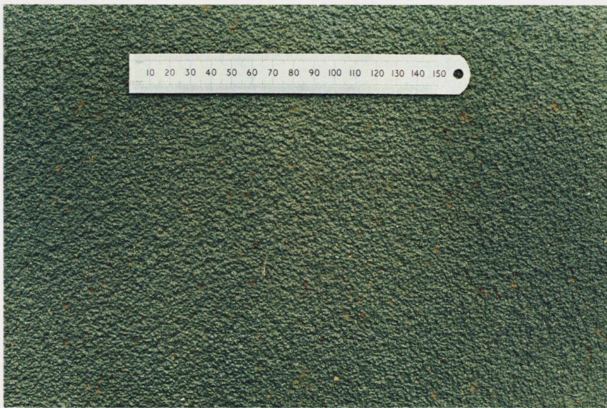
Figure 2 Sealcoat Green Deck Surface
